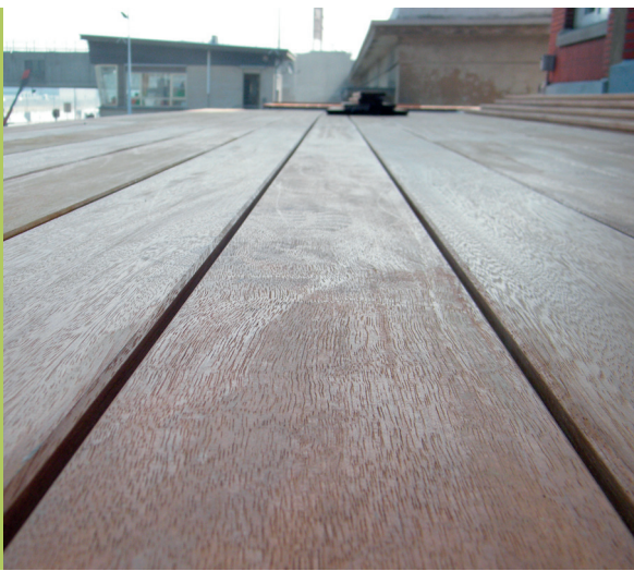
© FSC Belgium -Sluice of Ivoz-Ramet in FSC certified Afzelia
